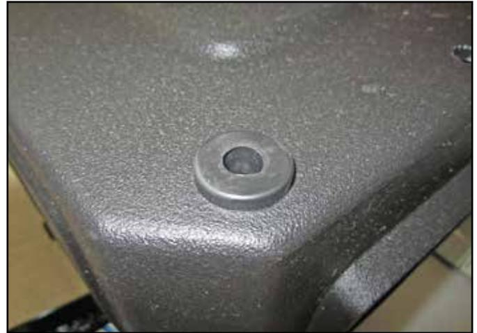
f. install the 784647 grommet into the larger left front mounting hole as shown.
